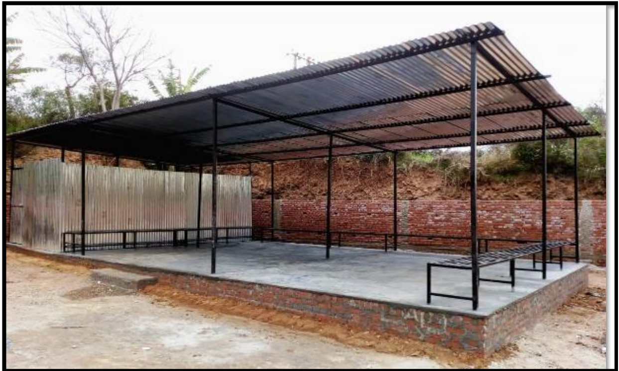
FEC Unit - Waiting area for mourners along with a store for fuelwood
