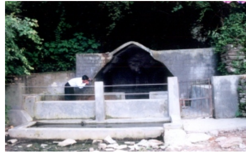
At this bawadi a gate prevents animals from soiling water meant for human use. Outside the gate an overflow tank can be used by livestock and other animals.
