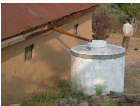
A pipe conveys rainwater collected on the building's roof to a filtration tank placed atop a ferro-cement storage tank.
