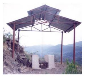
FEC reduces consumption of fuel-wood by 30% in cremation of a deceased and is an environmental friendly technique.
